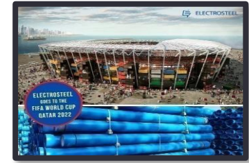
Ras Abu Aboud Stadium, Qatar
